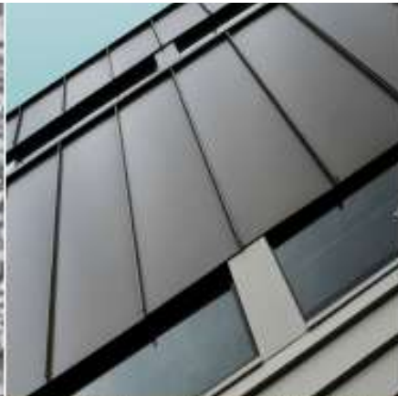
Walling and Eaves Colorbond Jasper Standing Seam
